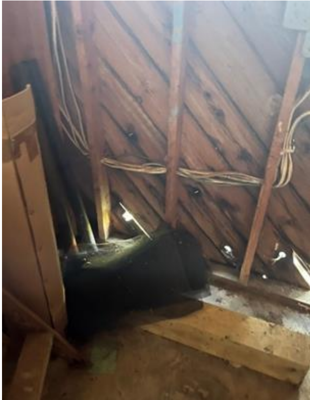
CONDITION OF SIDING
